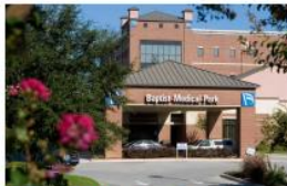
BAPTIST MEDICAL PARK – NINE MILE PENSACOLA, FLORIDA 850.208.6000
